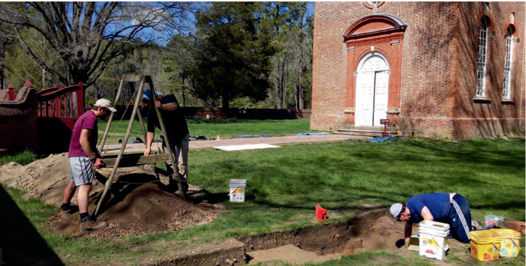
Churchyard Excavations Begin – Archaeologists began excavations in November 2021 at a low point in the southwest churchyard that floods during heavy rains. A catch basin here will collect water and transport it under the churchyard wall through a drainpipe that connects with larger drain lines running to an outfall point near a ravine behind the Chase Center administrative building.
