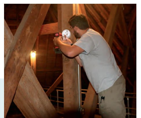
Derick Overstreet with ODCS Protection Systems in Warsaw installs a heat detector in Christ Church’s roof during a security upgrade in 2020.
