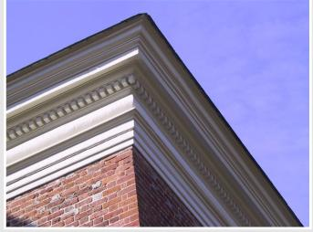
Preservation includes cleaning, lightly sanding, repairs to deteriorated woodwork, and painting with an egg-shell white determined by historic paint analysis to be the original color like that seen here following preservation work in 2002.
