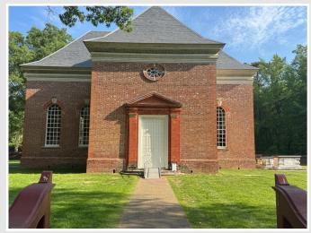
This view in May 2025 from the south gate shows how the buildup of dirt, mold and cobwebs on the entablature has discolored it compared to the doors and windows, which have been preserved in recent years.
