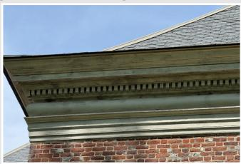
Mold, dirt and cobweb build up (April 2025). Note how the wood has become desiccated in areas.
