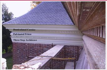
Fabricated of wood and standing four feet tall, the entablature's three-part design includes a denticulated cornice, pulvinated frieze and three-step architrave.
